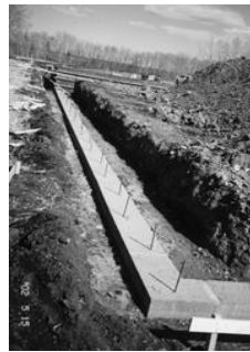
Construction begins April 2002.
