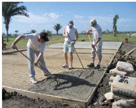
Pouring concrete for classroom.
