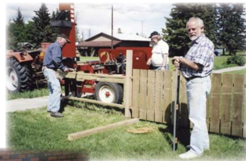
Fixing and painting the fence at Foothills Camp.
