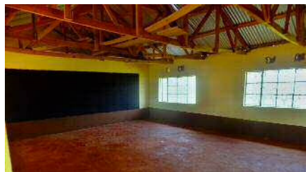
Inside one of the two new classrooms at Kisii Deaf School
